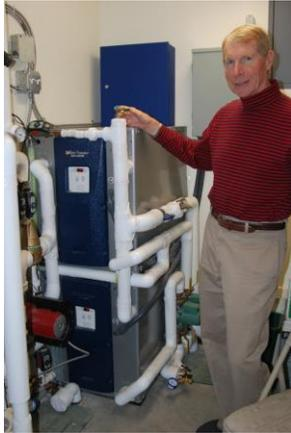
Caption: Dick Bourne shows off the equipment for the entire 3-story building: 2 geo-thermal (or ground-coupled) heat pumps and their connections to the radiant heating and cooling systems and the water storage tank.
