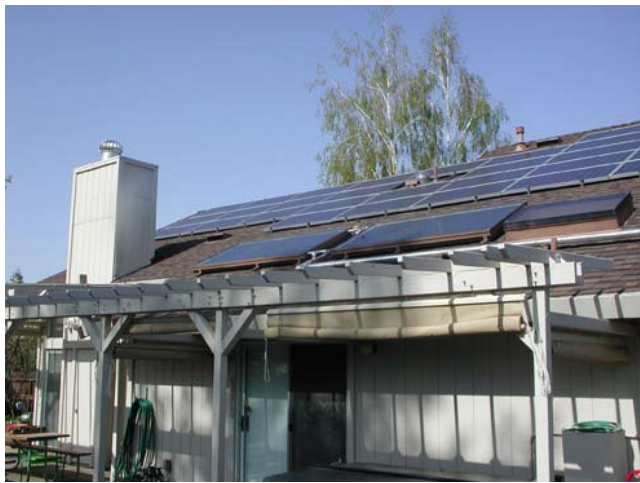
Alan Pryor supplies 100% of his electricity with his PV system. He is careful to shade the patio and south-east windows in the summer to keep the interior of the house cool.
