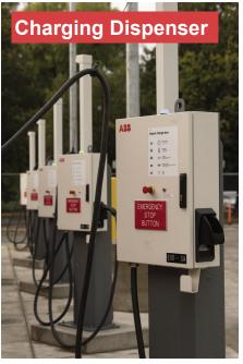
Unitrans currently has seven chargers serving 14 charging stations. The chargers are manufactured by ABB and provide 150 kwh per charger. Total charge time for two "empty"
